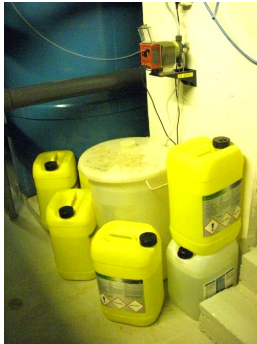
Figure 9: The dosing station of the flocculent at Husebybadet. The arrangement on the wall is the continual dosing machine.
