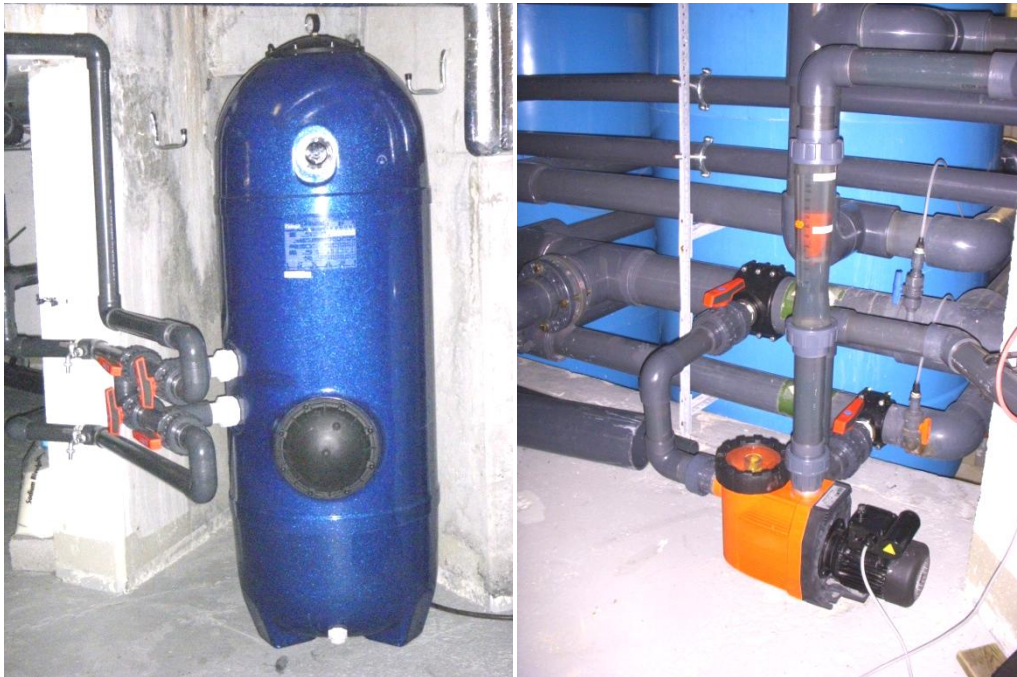
Figure 3: The glass filter used in the experiment installed at Husebybadet is shown in the picture to the left. The picture to the right shows the pump and the rotameter installed before the glass filter as a part of the pilot plant.
