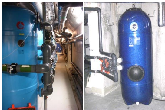
Figure 2: The sand filter is showed in picture to the left, while the glass filter is showed to the right.
