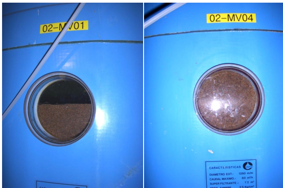
Figure 6: The picture to the left shows a correct filled sand filter, while the picture to the right shows a sand filter with too much sand.
