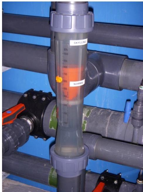
Figure 11: The rotameter installed prior to the glass filter, used for readouts of the flow values.
